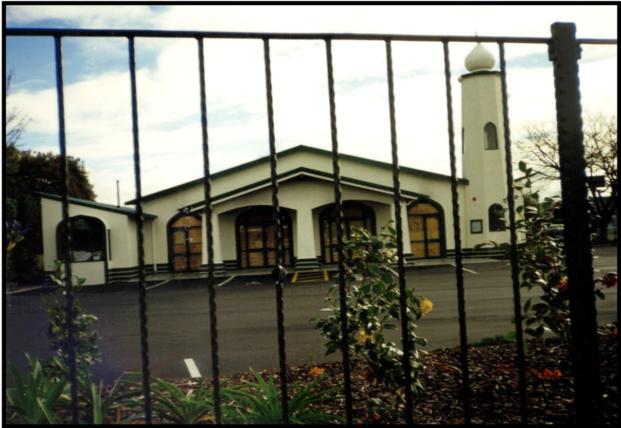
Figure 26: Hamilton Masjid restored to its original state by the middle of 1999.
