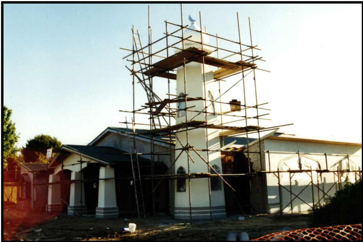
Figure 19: Construction of the Hamilton Masjid in progress, 1997.
